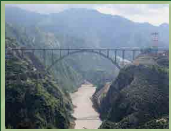
CHENAB RAIL BRIDGE
